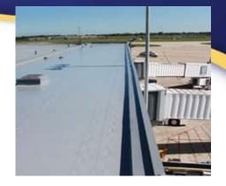
main corridor and in some of the vendor locations. Resulting damage was major and visible to airport travelers. There were also significant leaks in the communications room of the FAA tower. Temporary repairs by another contractor failed and roof replacement was now required. A full assessment of the roof, including core samples and an infrared moisture survey, identified saturated roof areas, as well as cracks in the roof penetrations and perimeter flashings.
