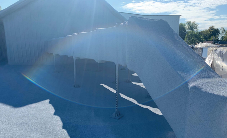
HVAC ducting encapsulated
