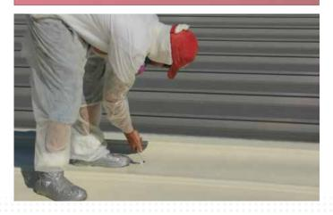
Systems decided to use CRFC's PremiSEAL 60R Roofing Spray Foam and SeamlesSEAL ULTRA HS Silicone Coating to complete this rooftop restoration.
