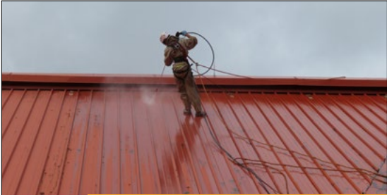
Power Washing Roof Surface
