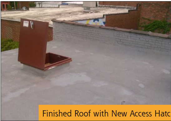
Roof Surface - After
