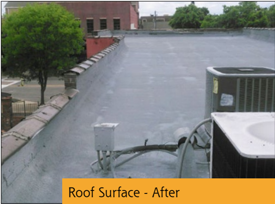
Roof Surface - After
